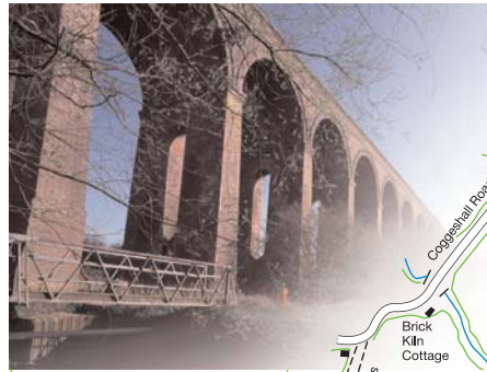
Chappel Viaduct, Chappel
